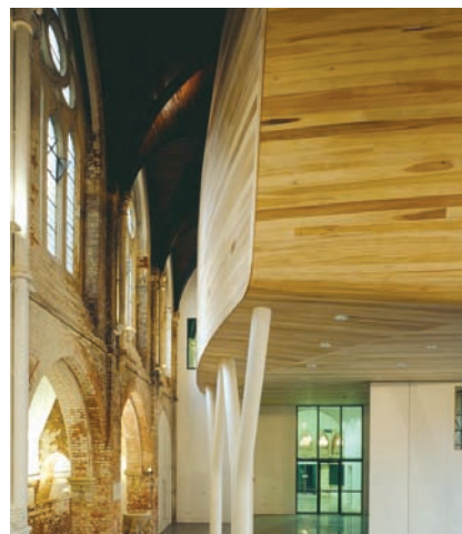
Right: Haberdashers' Hall, London. American white oak is used throughout. The ceiling diagonals are the top chords of the steel-tied roof trusses (see also back cover). Hopkins Architects. Engineer: Arup.
