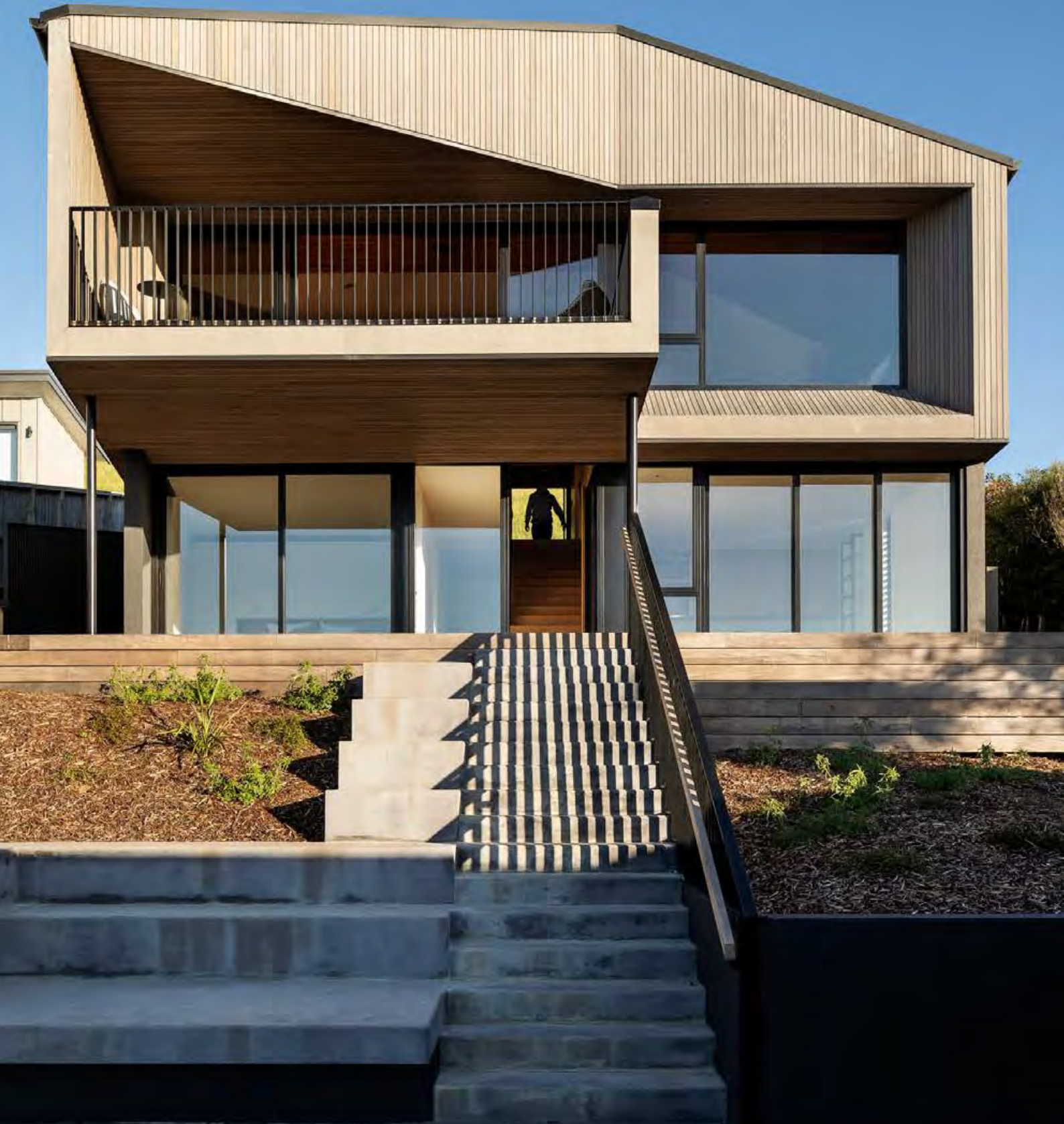
Picture: Western Red Cedar Cladding - Otamo Beach, Studio Brick Architects and Lloyd Hartley Architects
