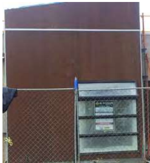
0 MONTHS: Recently built, this shows the beginning colour of Weathertex Natural boards.
