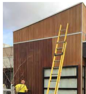
STAINING: Stain in the same direction that the boards run eg. Vertical for vertical cladding.
