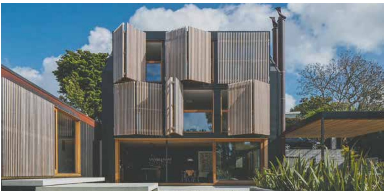
Western Red Cedar Fins, Location: Auckland Studio 2 Architects
